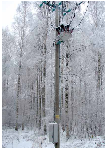
OSM RECLOSER AND CONTROL AND COMMUNICATIONS CUBICLE
